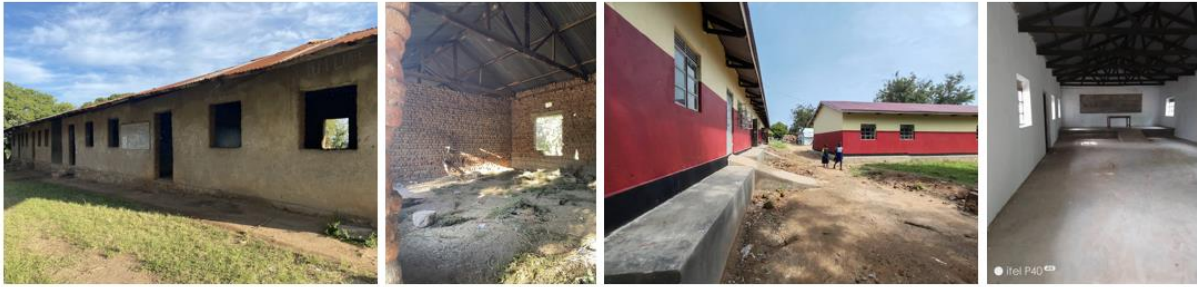
Situation before- and after the renovation completed
